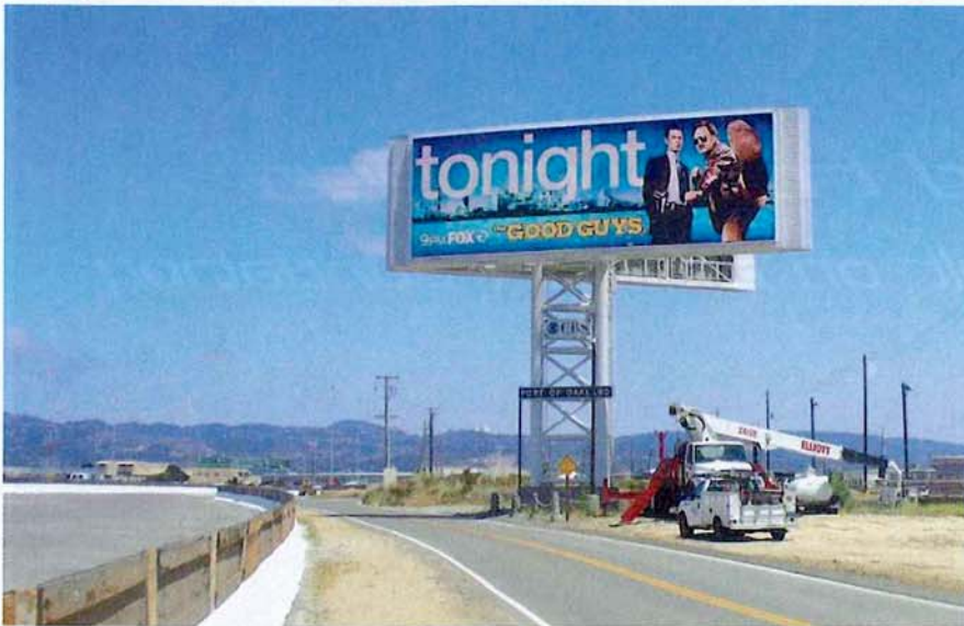
In the San Francisco Bay area, along the East Bay side of the San Francisco-Oakland Bay Bridge, CBS Outdoor erected a 20 x 60-ft., double-faced, digital billboard. Because of the heavy traffic and the LED-cabinet weight, the billboard's sign structure was custom designed for road placement on the East Bay side of the bridge.
