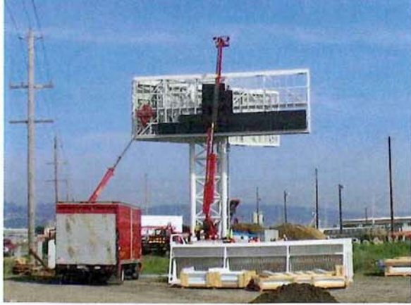
In the San Francisco Bay area, along the East Bay side of the San Francisco-Oakland Bay Bridge, CBS Outdoor erected a 20 x 60-ft., double-faced, digital billboard. Because of the heavy traffic and the LED-cabinet weight, the billboard's sign structure was custom designed for road placement on the East Bay side of the bridge.
